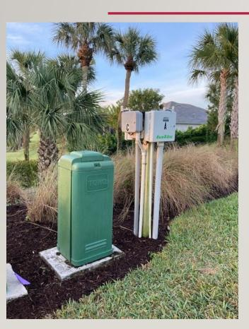
7/2/25- Request from GulfScapes to troubleshoot this satellite. Found a blown 8-amp common fuse and replaced the fuse at no charge.
