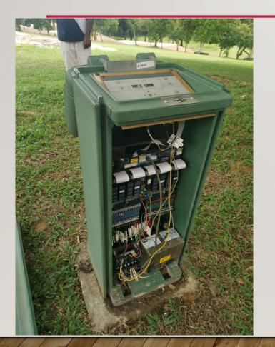
Satellite I-3 Bent Creek – Satellite failing to communicate. Performed investigation and identified failing power switch, radio modem and faceplate. Replaced failing components. Invoice directed to CDD.
