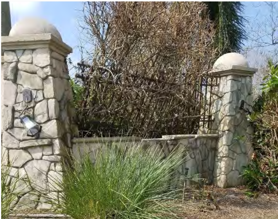
South Monument Sign (Right-Hand Railing and Cap Damage)
