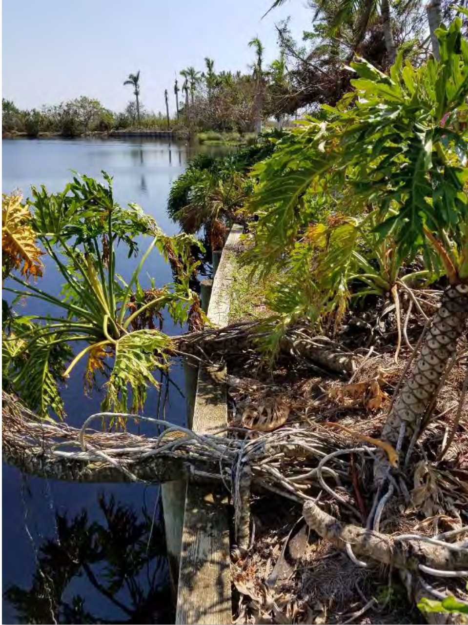
South Bulkhead (behind end of southern wall) Heaving towards lake and some wash-out of backfill observed.
