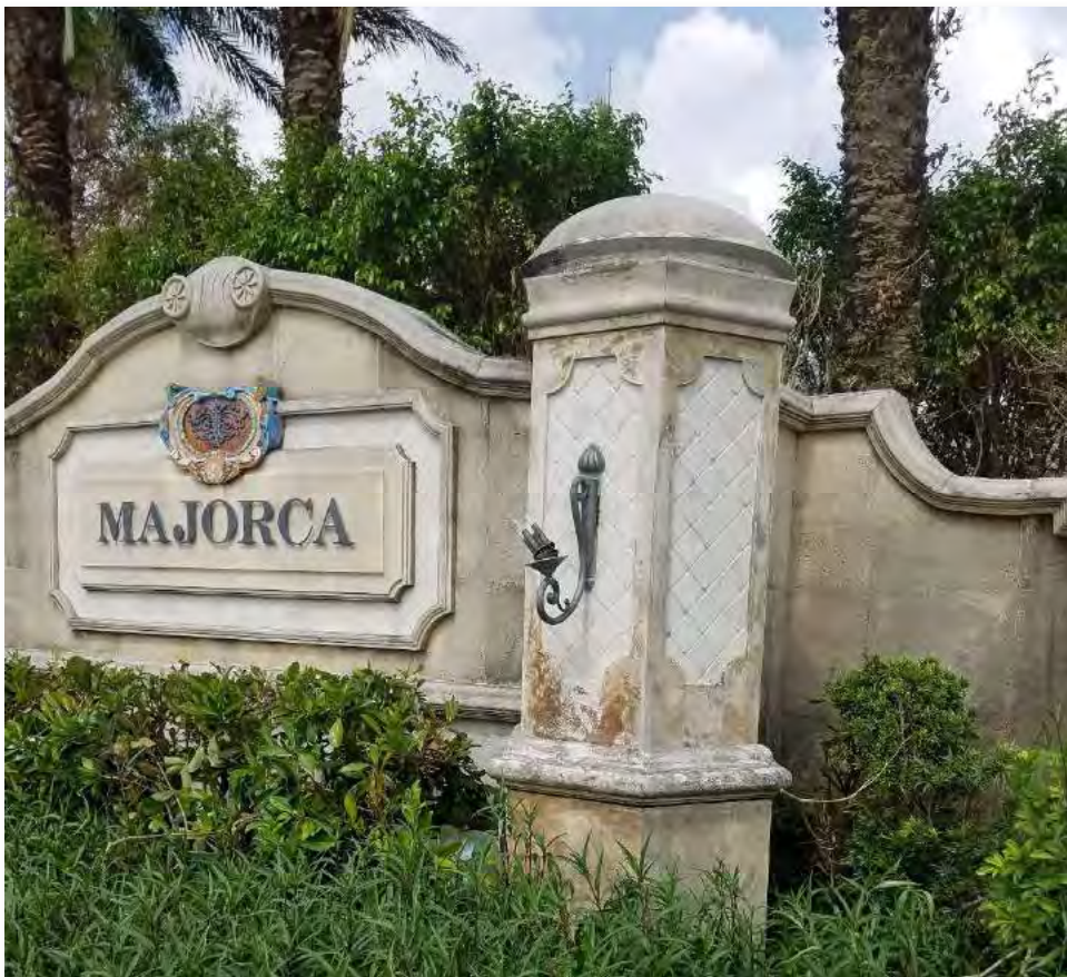
North Monument Sign (Light Fixture Damage)
