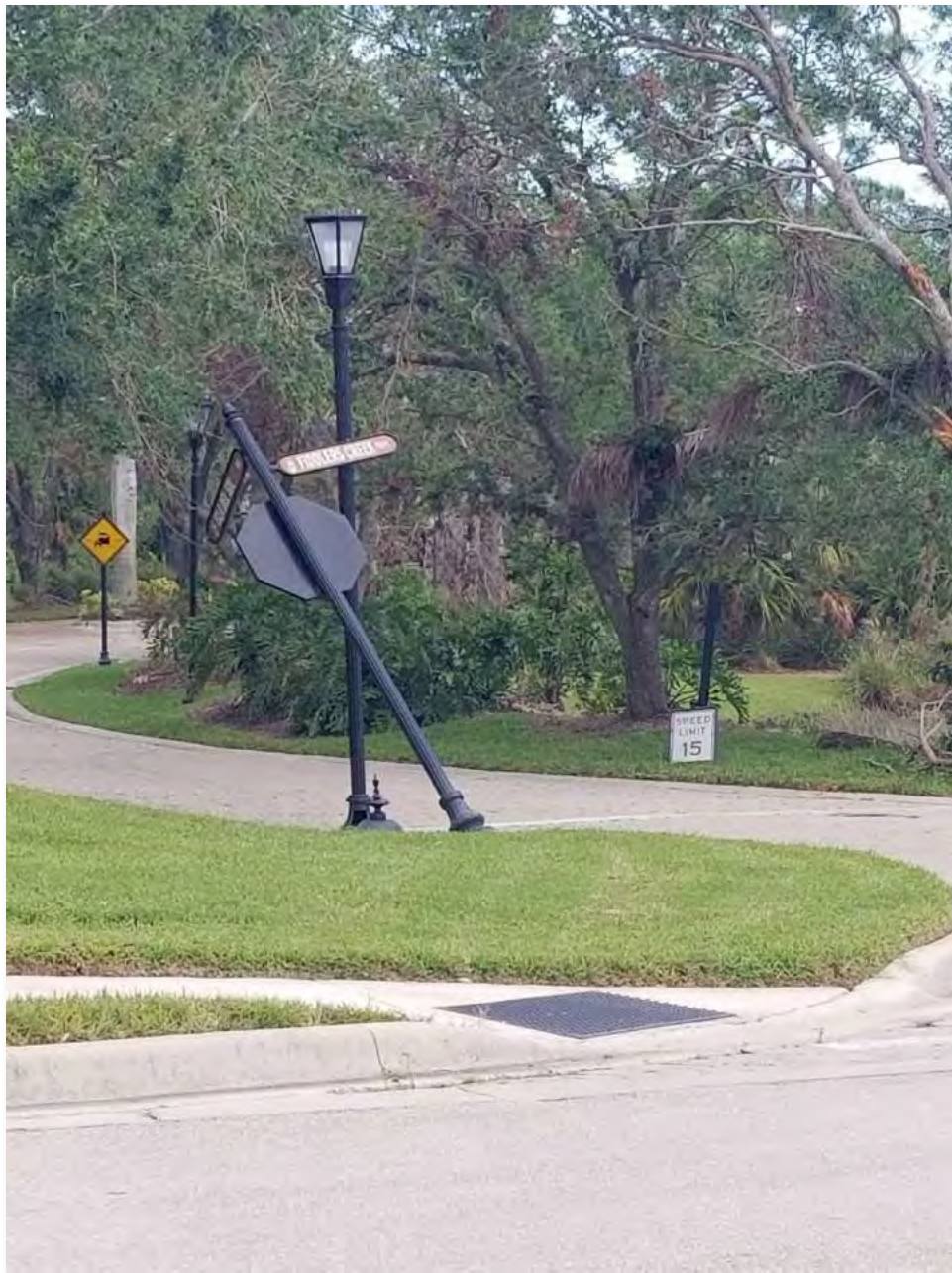
Typical Bent Decorative Street Sign (Combination Stop Sign and Street Name) Typical Broken Decorative Sign (speed limit sign in background)
