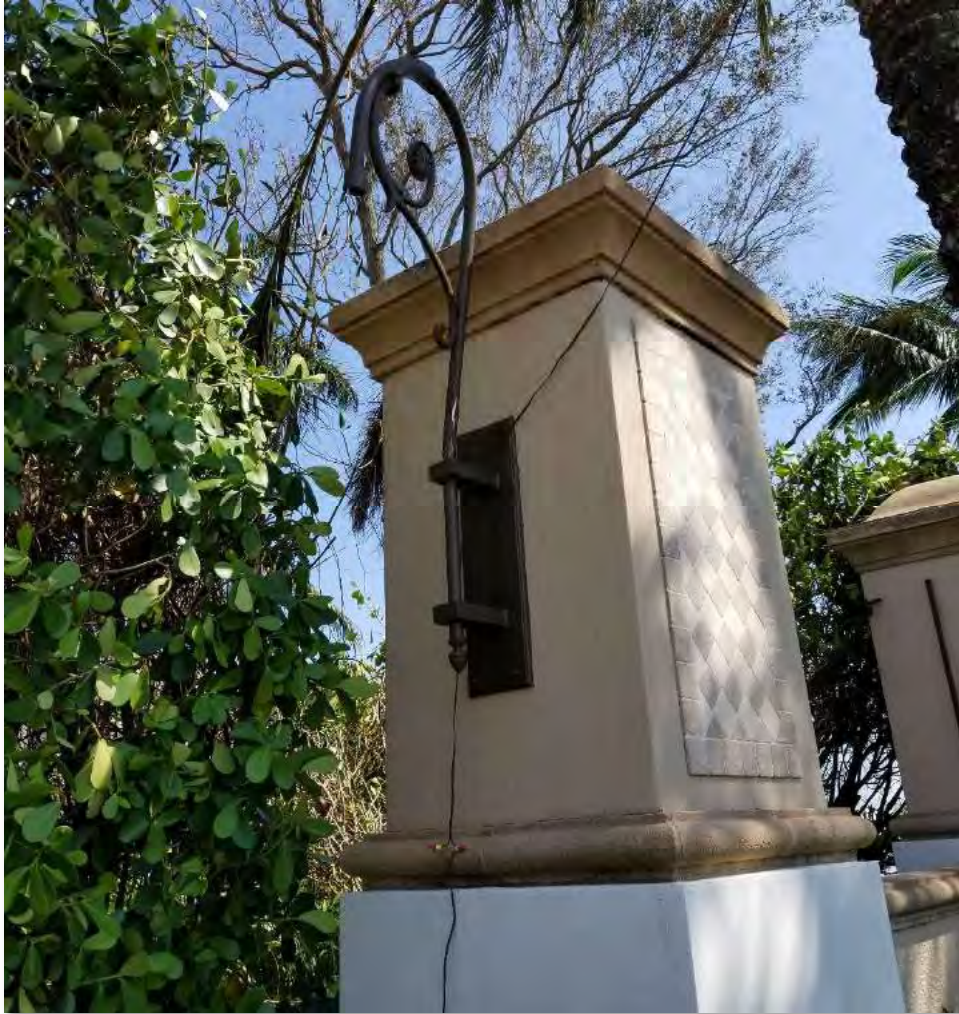
South Monument Sign Left End Lighting Fixture Missing
