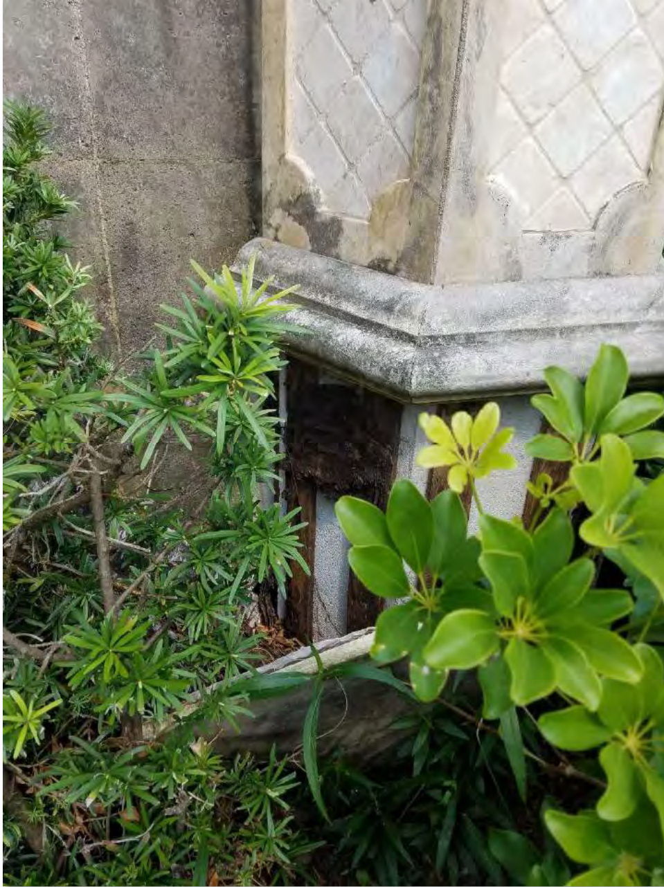
North Monument Sign (Bottom Left Façade Damage)
