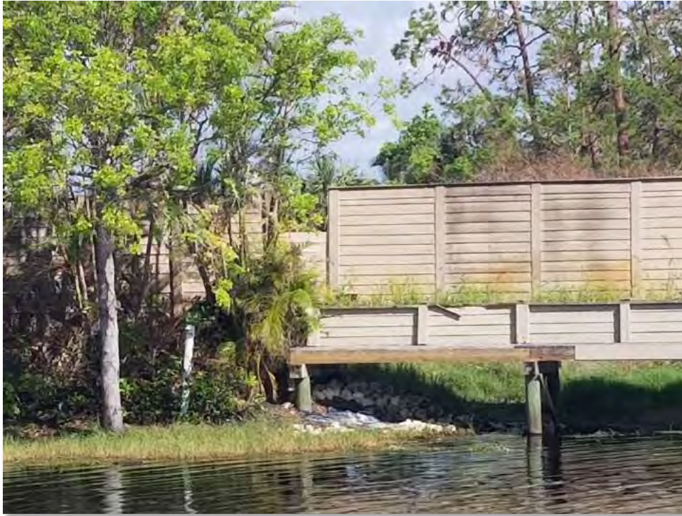
Aviamar (Damage to horizontal panels, planter box, and exterior siding on cap board.)
