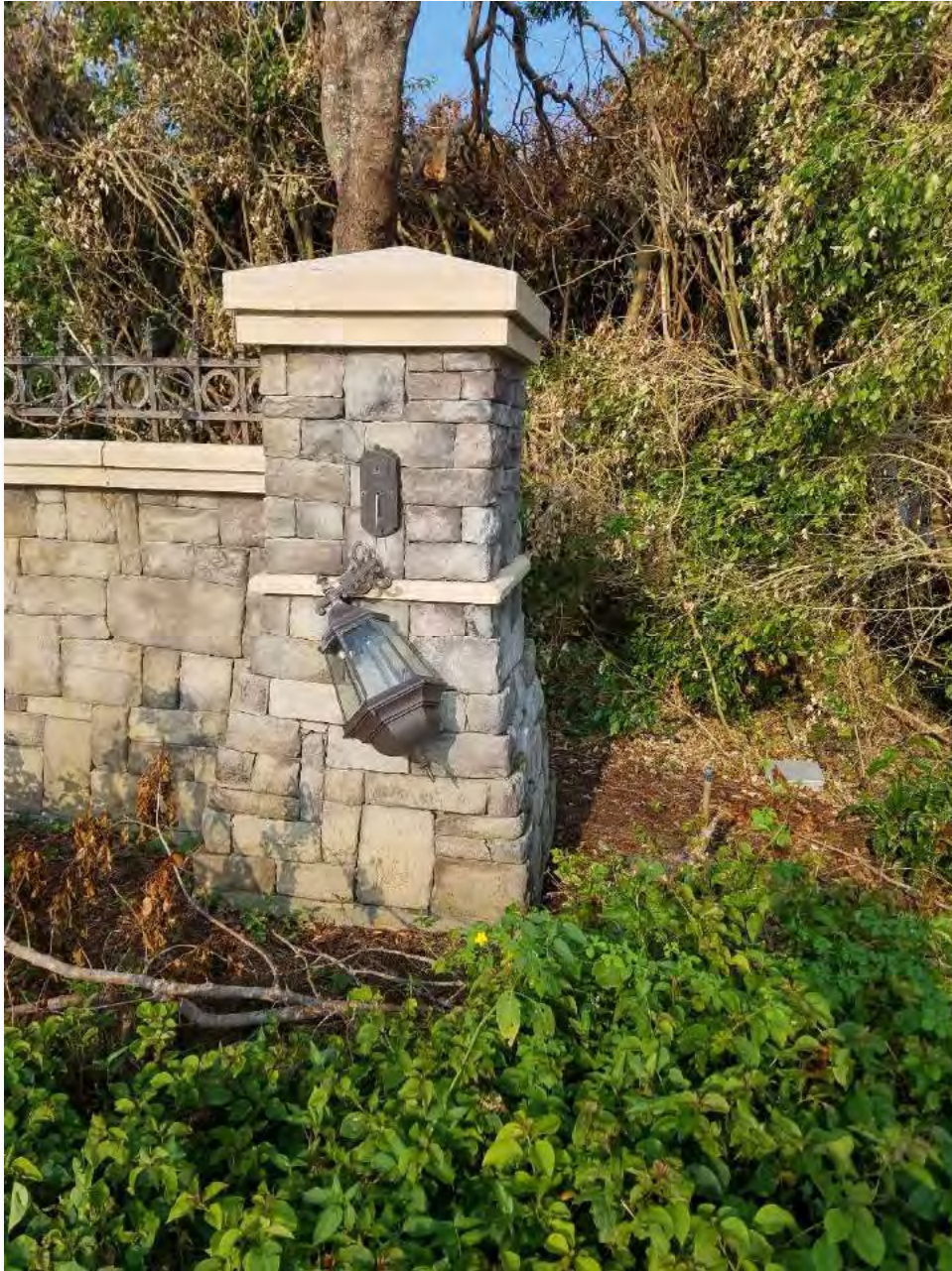
Damaged Light Fixture Right-Hand Side
